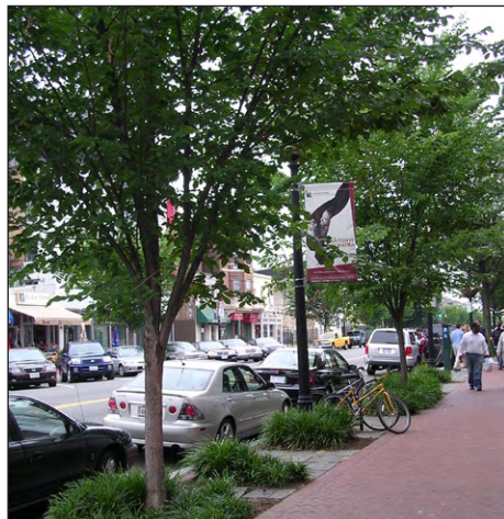
Trees on 8th St., SE are growing in structural soil with permeable pavers covering portions of the tree space.
